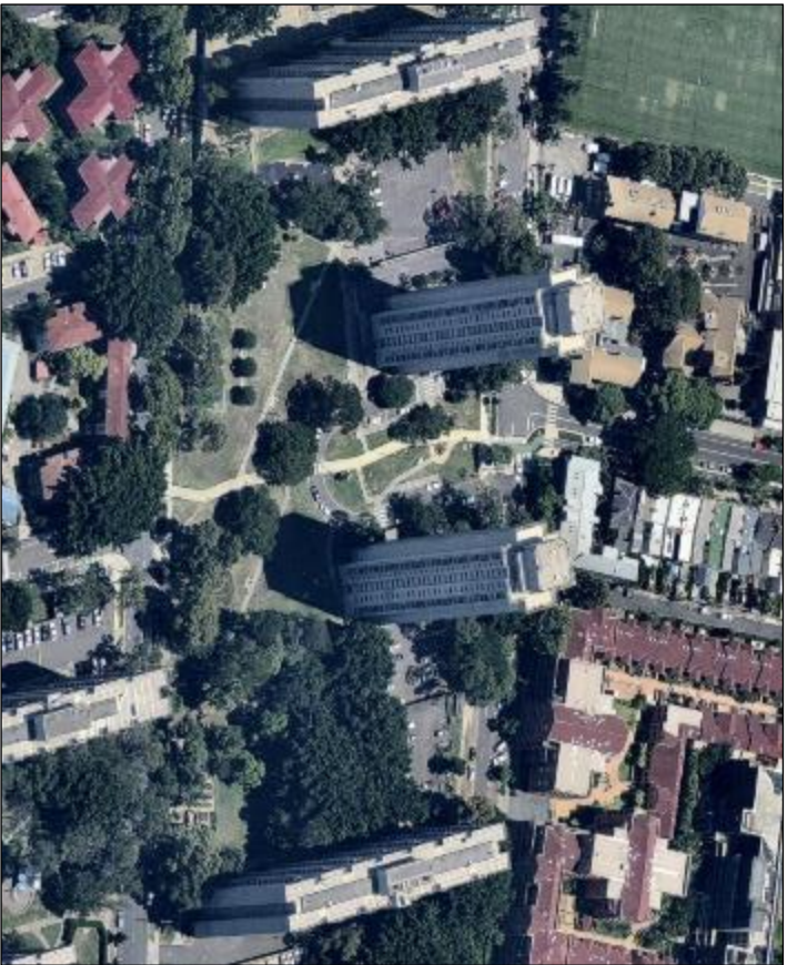
Figure 3-12 Tower development in the northern part of the Precinct. (Source: Nearnmap)
